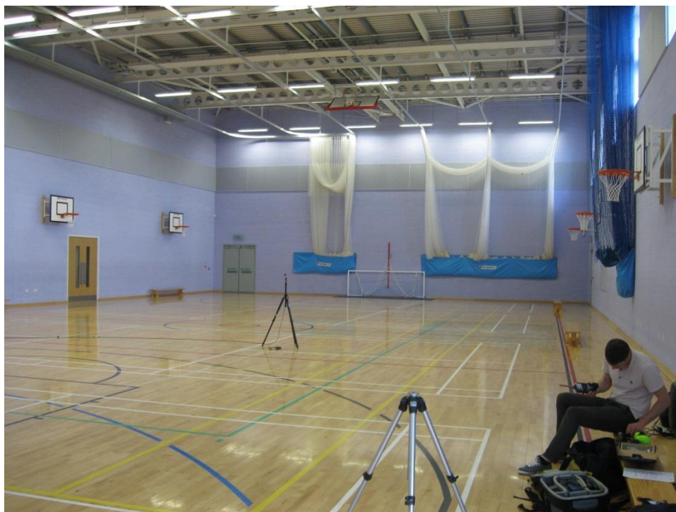
Figure 1: Hall 1, with the band of grey absorbent panels visible at high level
