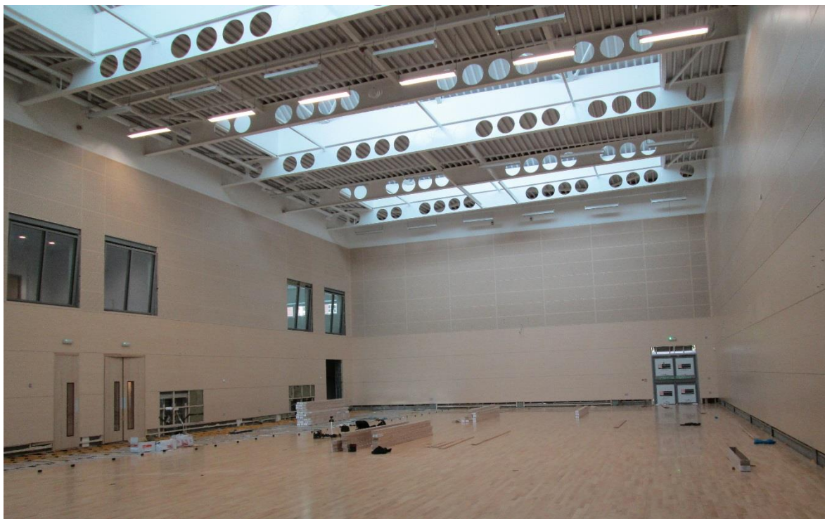
Figure 2: Hall 2, with perforated panels visible above 3 m height around all sides
